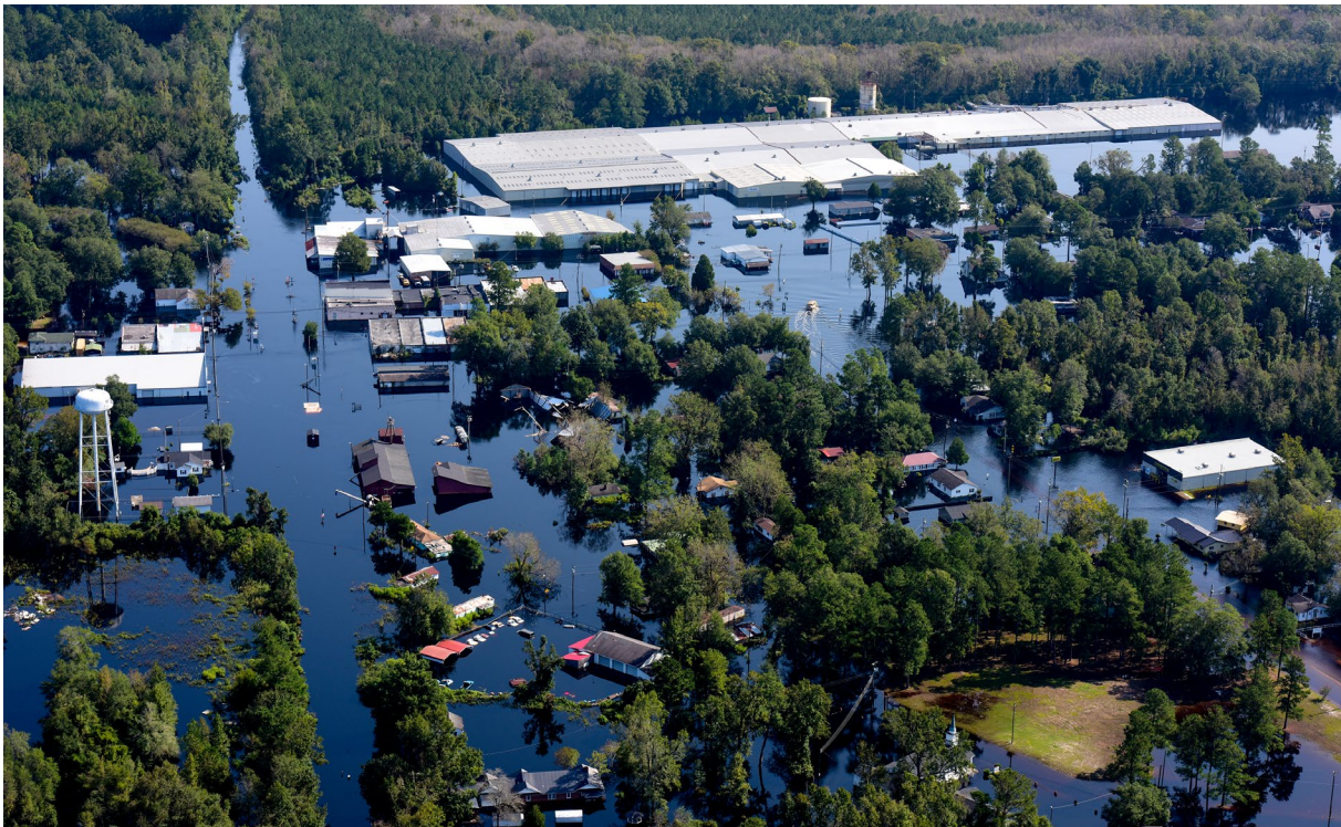
A flooded area of South Carolina due to Hurricane Florence in 2018. (South Carolina Air National Guard)
