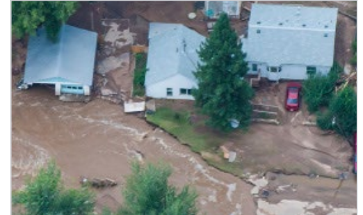
Boulder County Flooding Source: US National Guard
