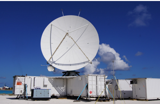
Fixed Ground-based Radar :: detecting cloud particles and winds
