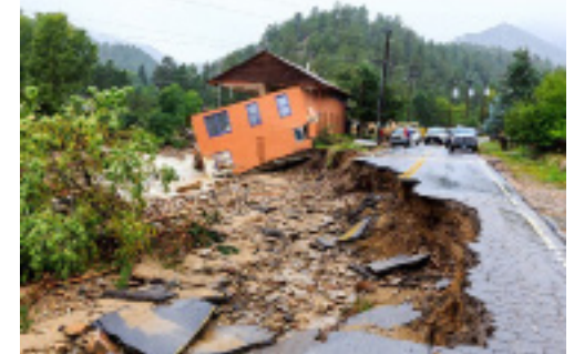
Boulder County home destroyed by flooding
