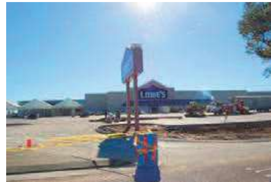
CH7-42: Stormwater facilities under construction.
